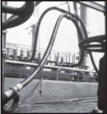
Typical ship to shore loading/unloading flexible piping system
